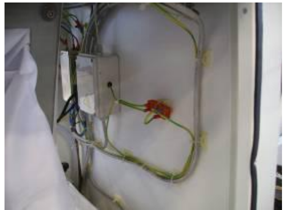
Ground connection during maintenance operation
